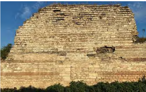
Fig. 2- An example of the historical stratification of the walls, displaying different construction periods and a closed postern (3 rd secondary gate), at the main wall MW_42-43 (1)
