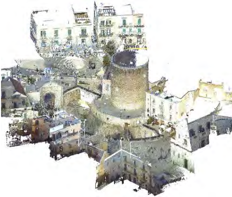
Fig. 3- Point cloud of the whole complex (graphic elaboration by the authors, 2025)
