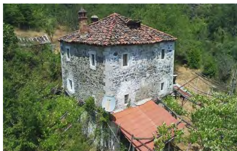
Fig. 3- Aerial view of the kulla house (source: the authors)
