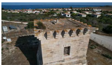
Fig. 1- View of the Tower in the landscape
