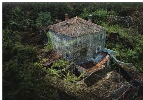
Fig. 5- Close view of the dense point-cloud (source: the authors)
