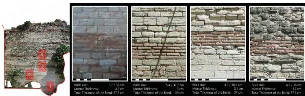
Fig. 10- An example of masonry measurements taken from the west façade of MW_56-57
