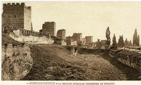
Fig. 1- A historic postcard depicting the state of all three layers of defence of the Land Walls; the main walls, outer walls and the ditch (source: İBB Kütüphane ve Müzeler Müdürlüğü Koleksiyonu, Inventory no: Krt_077997_01)
