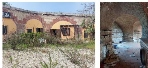
Fig.4- Forte Scrivia. Main building, which housed a restaurant until 2020, with the inner courtyard and rooms severely damaged
