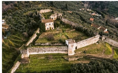
Fig. 2- The Rocca di Sala in Pietrasanta (aerial photo by Andrea Crudeli, 2024).
