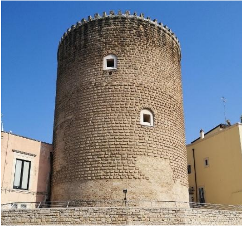
Fig. 2- View of the restored tower (photo by the authors, 2025)
